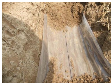
Installation of subsurface water retention membrane
